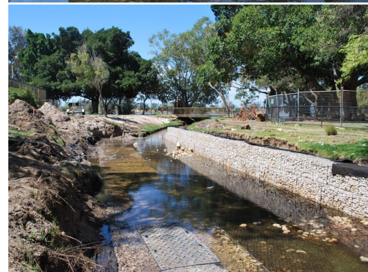
▲ March 2014: Installation of gabion wall
