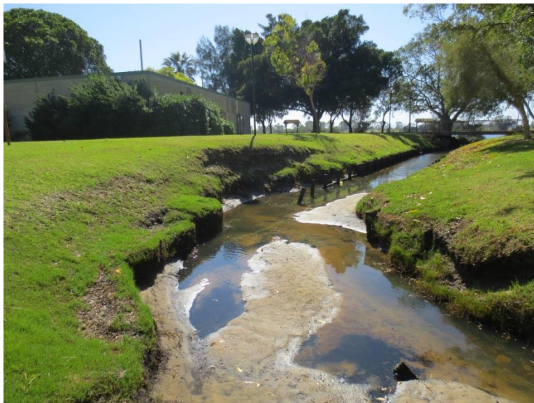
▲ October 2013: Initial site conditions
