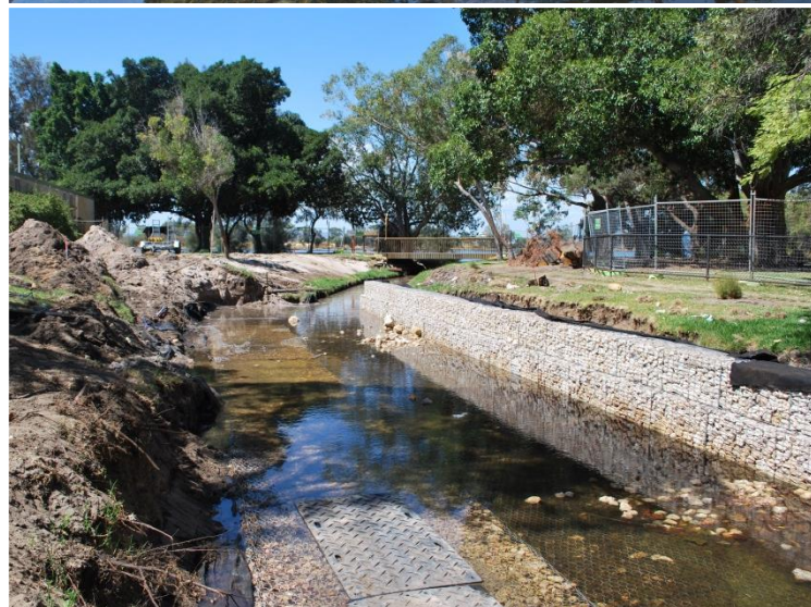
▲ March 2014: Installation of gabion wall
